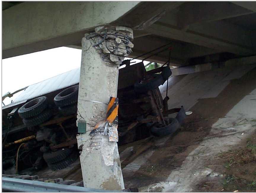
Figure 8. Photo. MnDOT Example of Column Damage Due to Truck Impact.
