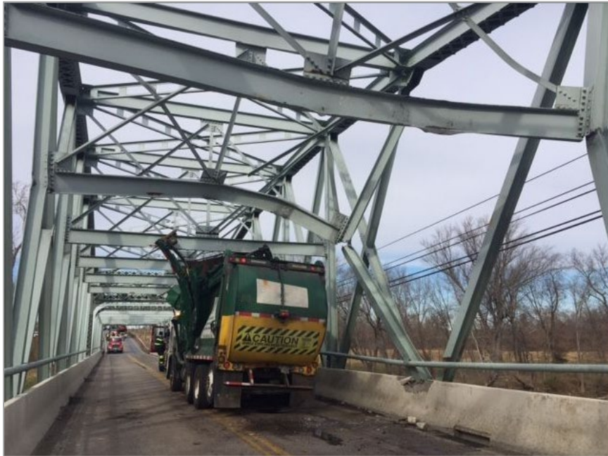
Figure 12. Photo. MSHA Example of Steel Truss Damage Due to Garbage Truck Impact.
