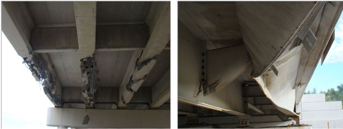
Figure 6. Photos. MDOT Examples of Typical Type III Damage.
